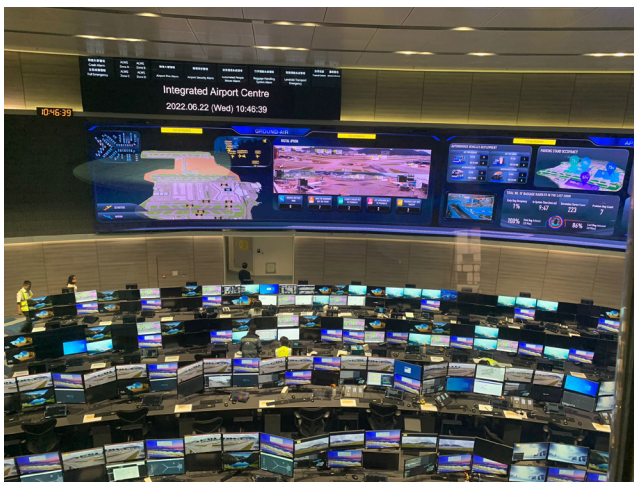
Hong Kong International Airport, Integrated Airport Centre (IAC)
